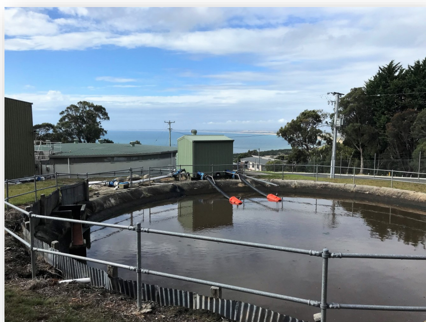
Photos: Bridport Water Plant and
